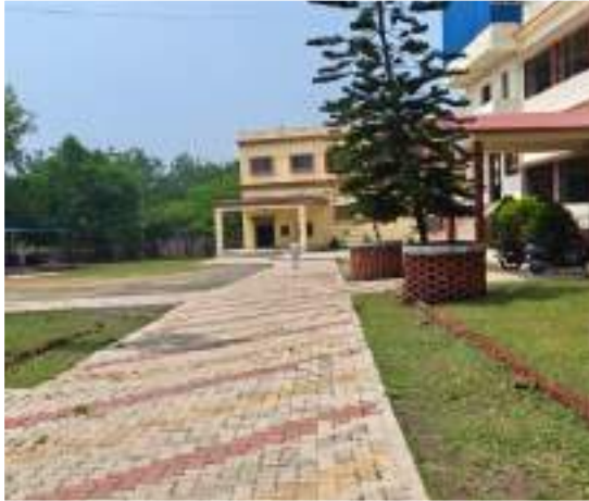
Paving Stone Installed In Campus
